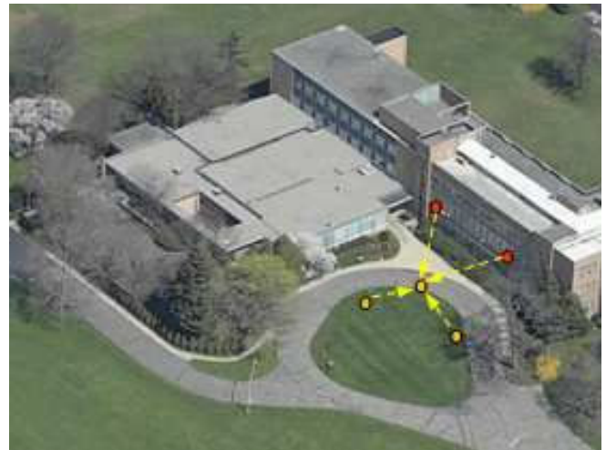
Fig. 5. Static anchor node locations in the map are shown in red corresponding to radios placed on window sills on the second floor of the building. Mobile nodes attached to backpack systems worn by three users during live exercise are shown in yellow.
