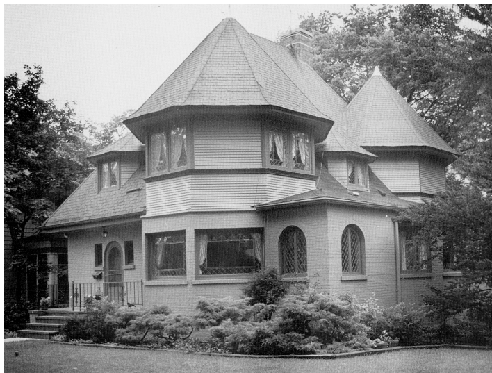
Figure 13. Transition house: Wright's Emmond house, LaGrange, Illinois (1892)
