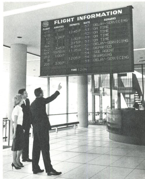
In March 1962, the Flight Information Board as shown above was installed in the Western Airlines Terminal Building in Los Angeles, California, and comprised 300 characters of the self-encoding type.
