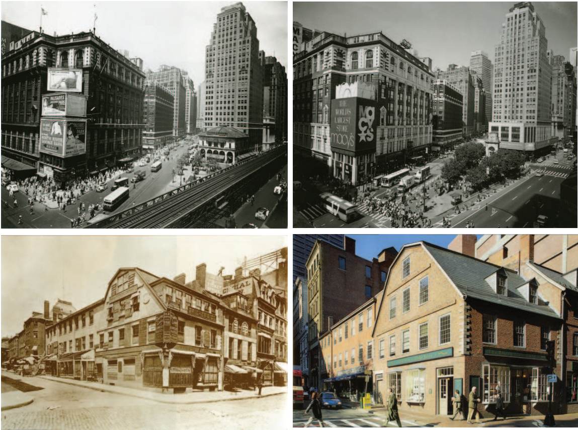
Figure 2-6: Rephotography gives two views of the same place around a century apart. Pictures are from New York Changing [2] and Boston Then and Now [3].
