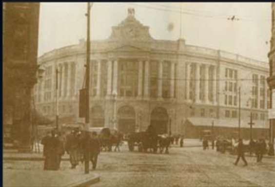
Historical Image of Boston Station
