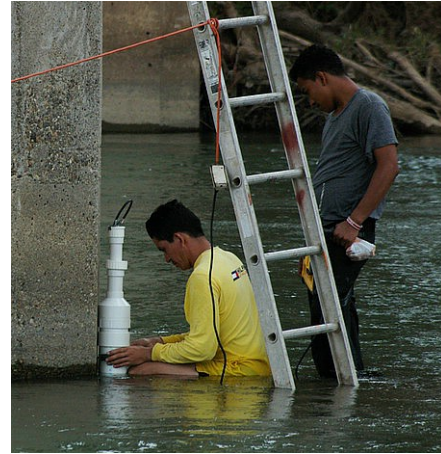
Figure 15. Installation of Water Level Prototype
