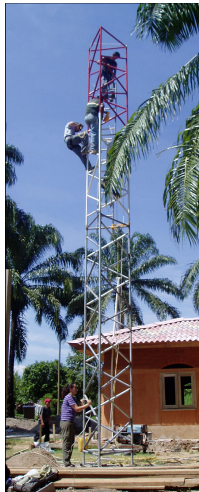
Figure 14. Installation of 10 Meter Tower at Office
