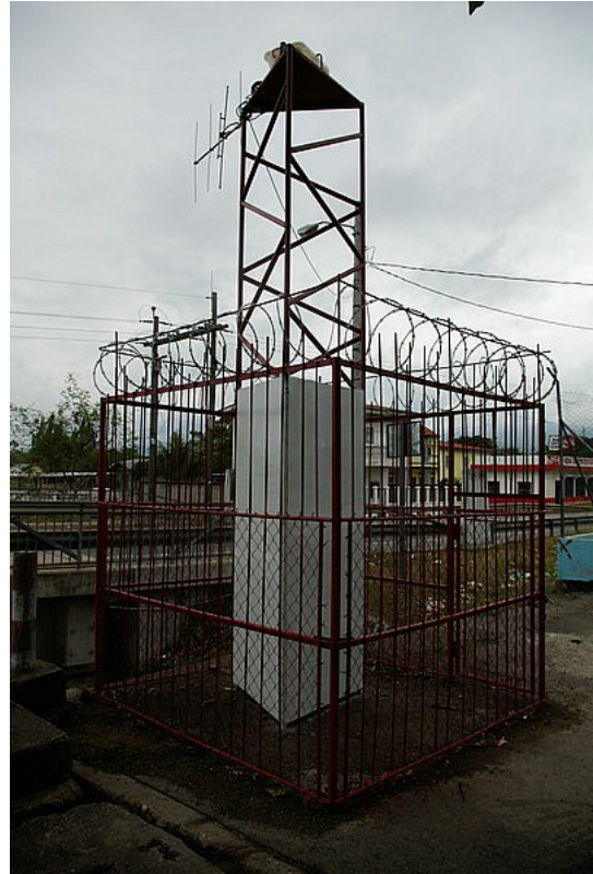
Figure 7. 5 Meter Antenna Tower for Computation Nodes
