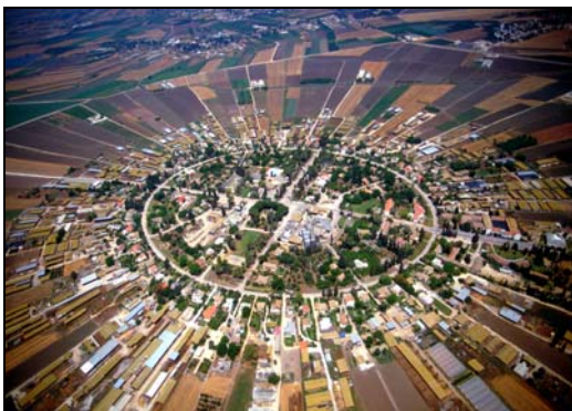
Figure 1. Aerial view of Nahalal village.
