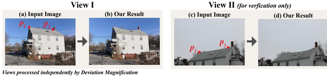
Figure 5.1: Revealing the sagging of a house’s roof from a single image. A perfect straight line marked by  $p_1$  and  $p_2$  is automatically fitted to the house’s roof in the input image (a). Our algorithm analyzes and amplifies the geometric deviations from straight, revealing the sagging of the roof in (b). View II shows a consistent result of our method (d) using another image of the same house from a different viewpoint (c). Each viewpoint was processed completely independently.
